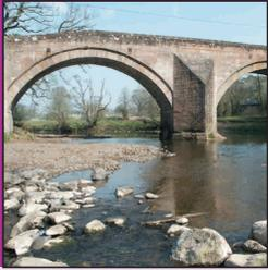
Stair Bridge was built in 1745. A few years later it was reported that the bridge had 'failed in its foundations.' In order to strengthen the foundations, old milestones that had recently been replaced with new stones were used to give protection to the central piers.
